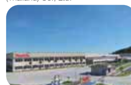
Thailand Makita Manufacturing (Thailand) Co., Ltd.
